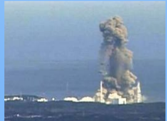
March 14 th , 2011 | Explosion of Unit No.3 in Plant I
